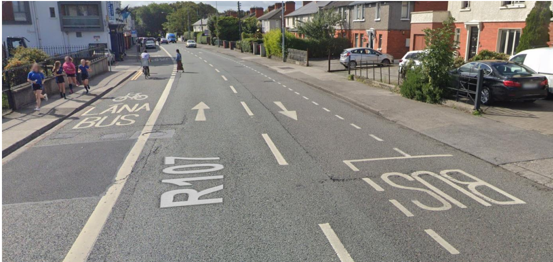
Figure 7-5: Localised Poor Road Pavement Condition on Malahide Road Near Junction with Crescent Place ©2019 Google Maps
