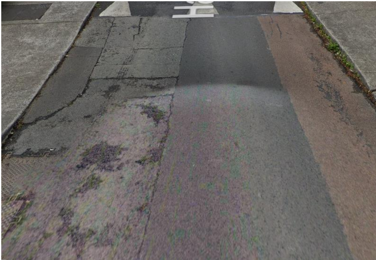
Figure 7-6: Localised Poor Road Pavement Condition on Haverty Road (Proposed Quietway) ©2021 Google Maps
